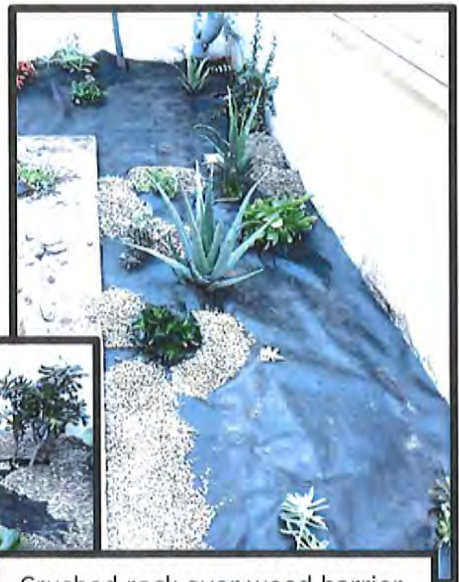
Crushed rock over weed barrier
